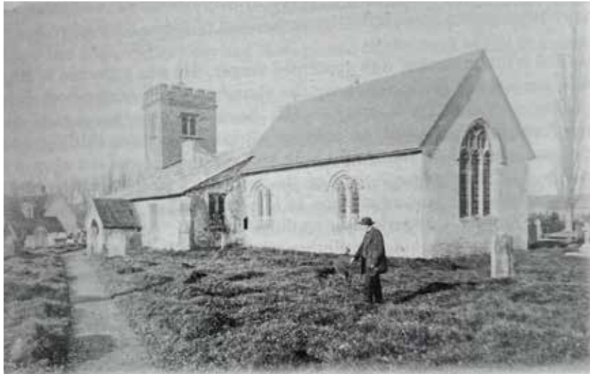
St Leonard's prior to the demolition of the tower and with its lowered nave roof in 1885.
