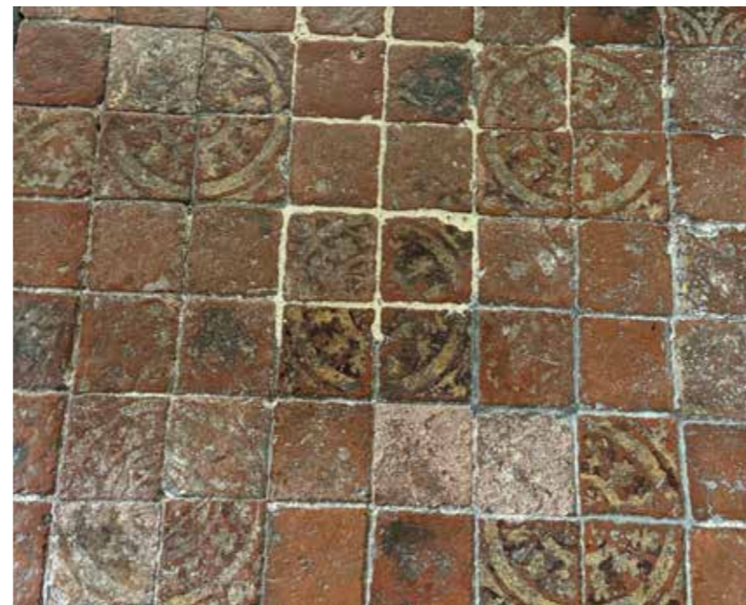
Chancel and sanctuary are tiled with medieval floor tiles red in the main with white slip patterns in places.
