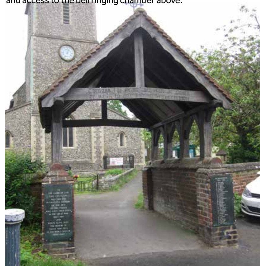
Erected in 1920 St Leonard's Lych gate is a memorial to the men of the parish who served in the great war 1914-1918.
